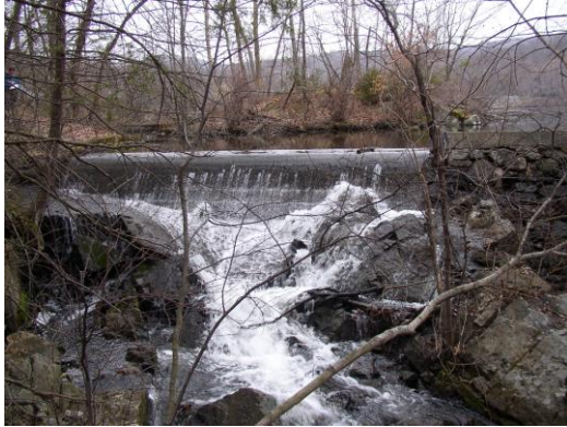
Westchester Lake Dam Primary Spillway
